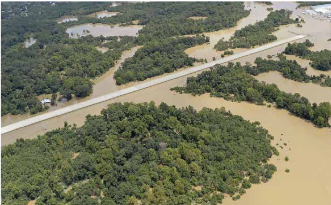
Flooding around the Magnolia Bridge in East Baton Rouge Parish.
