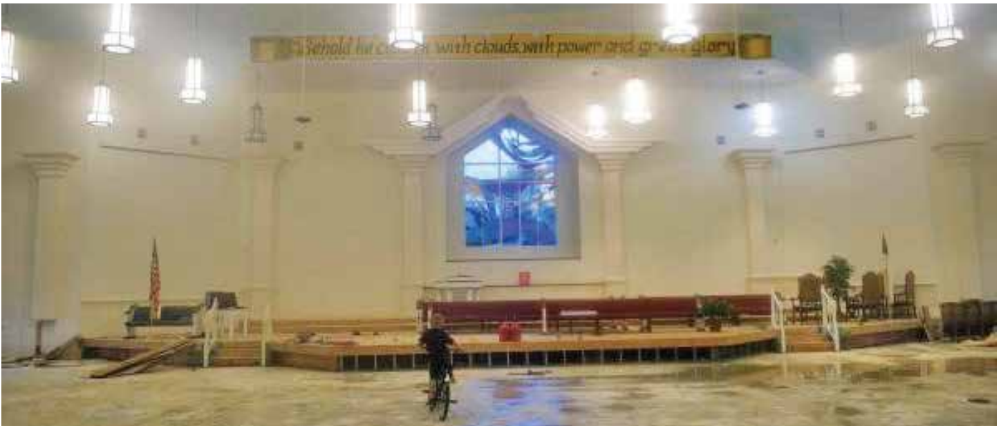
The Life Tabernacle Church in Baton Rouge was initially opened as a shelter for displaced residents. The church had to be evacuated just a few hours later when it began taking on water as well.
